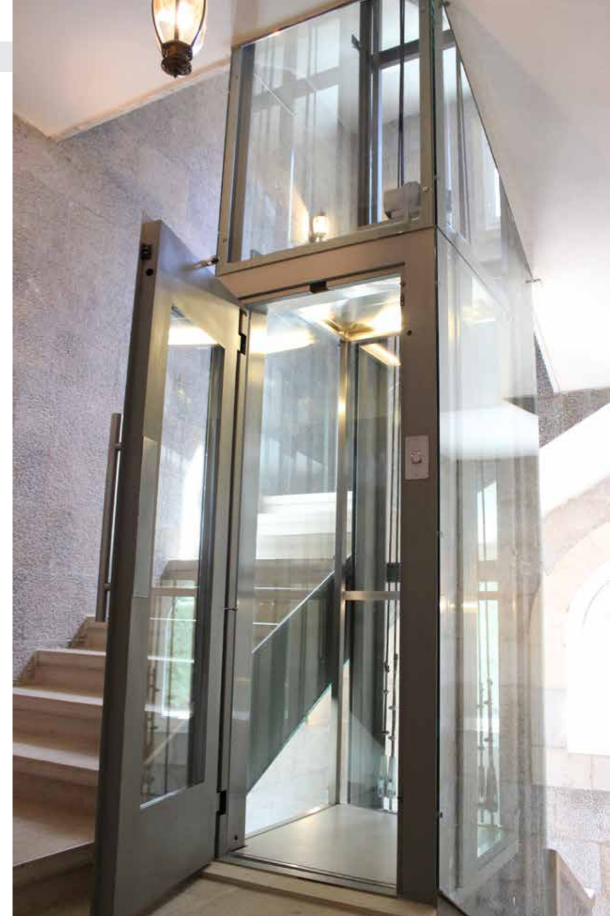
Residential Buildings Hydraulic Lifts Samaha Group (5 floors building) Location : Khenchara, Lebanon 2008
